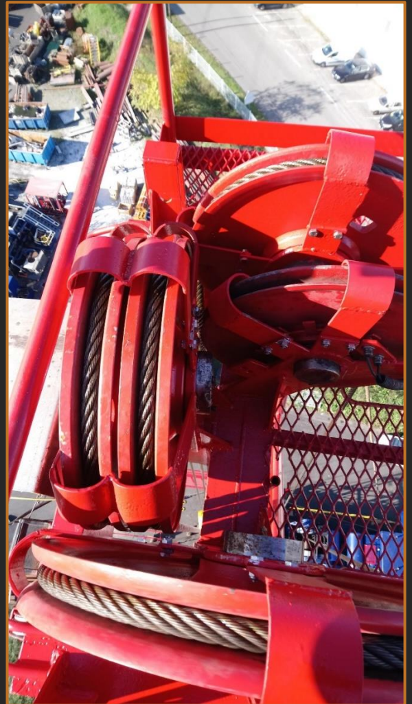
Maintenance quinquennale foreuse appareil de forage (RIG work-over)
